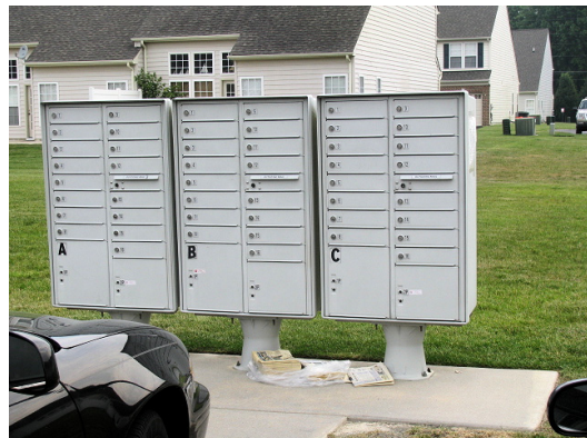
Typical cluster mailbox and concrete pad.
