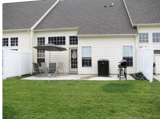
Typical rear elevation of townhouse unit
