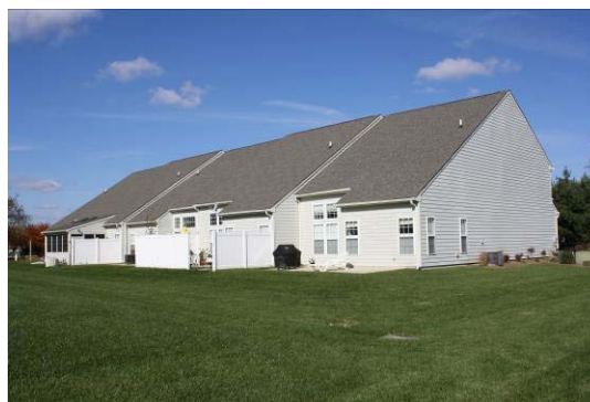
Rear of townhouse unit
